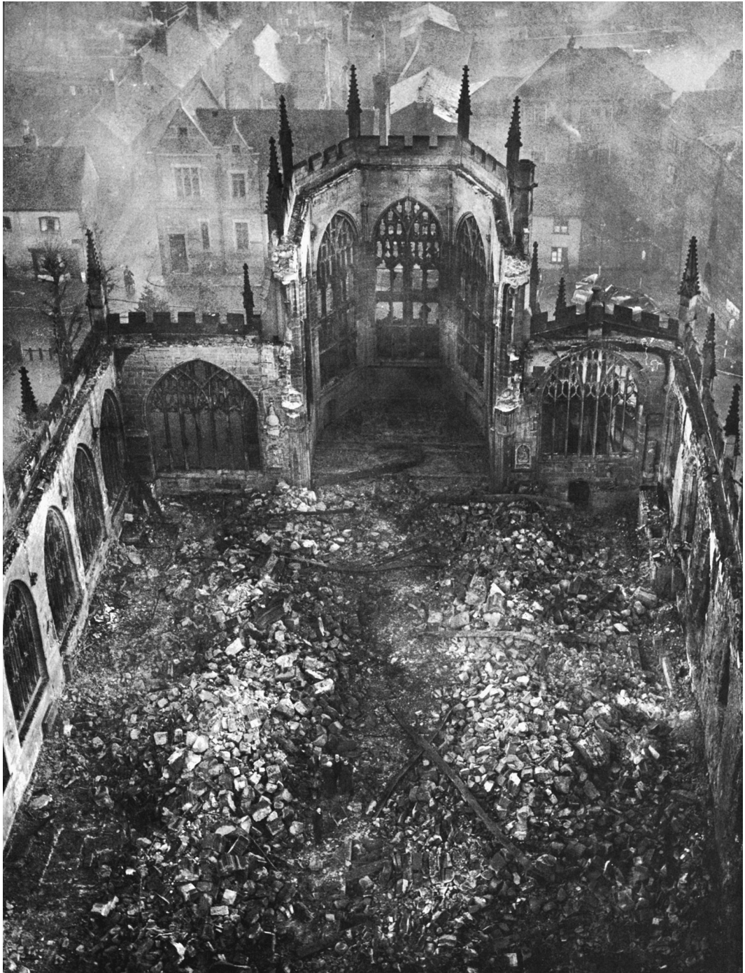
Fig. 12.1 Coventry Cathedral reduced to rubble by German air raids (November 14, 1940)
